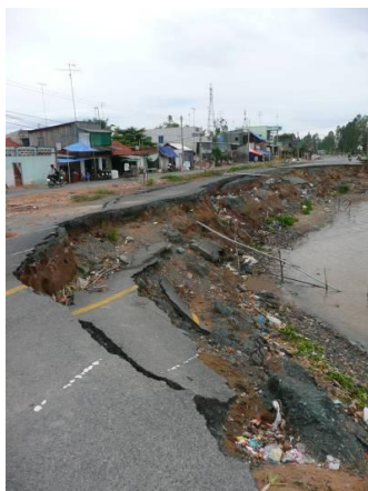
VISIT STUDY SITE – RIVER BANK EROSION – AN GIANG PROVINCE, MEKONG RIVER DELTA
