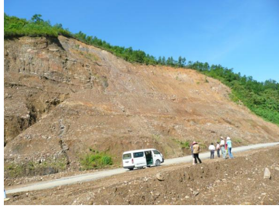
VISIT LANDSLIDE RISK AREA AT STUDY SITE – DONG GIANG DISTRICT, QUANG NAM PROVINCE
