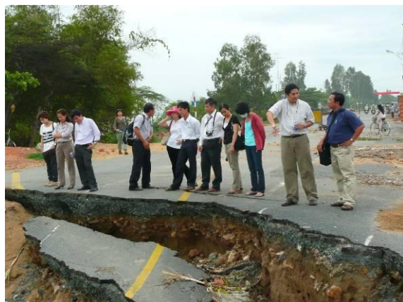
VISIT STUDY SITE – RIVER BANK EROSION – AN GIANG PROVINCE, MEKONG RIVER DELTA
