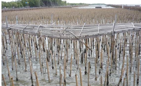
PHOTO 3: MANGROVE COASTAL PROTECTION AT THE MARINE AND COASTAL RESOURCES RESEARCH CENTRE (SAMUT SAKHON)
