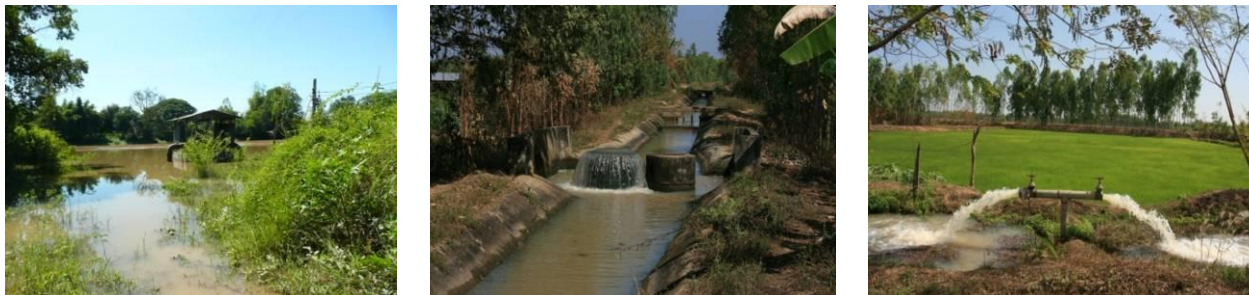
Figure 16: Existing pump station and water distribution system in Lao-oi District
