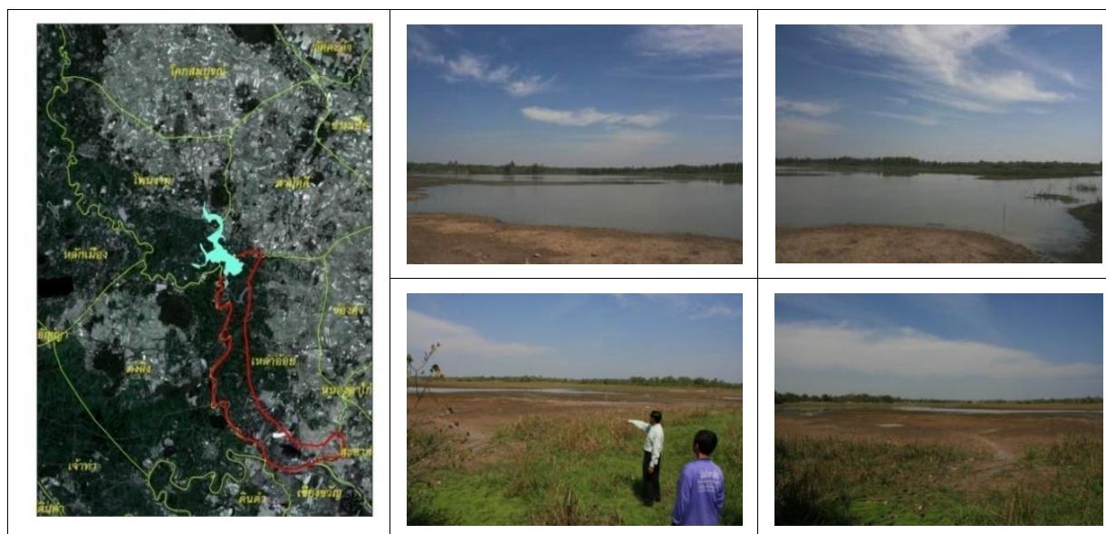
Figure 8: Natural reservoir in Lao-oi district that could be used to store water from flood season for irrigation in dry season.
